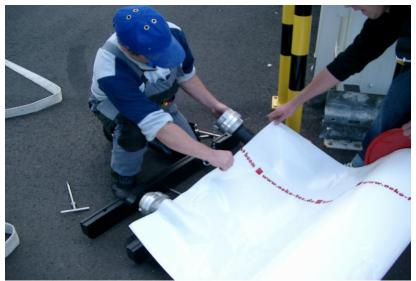
Place filling plugs into the boom chambers and press the plug firmly into the seats.
