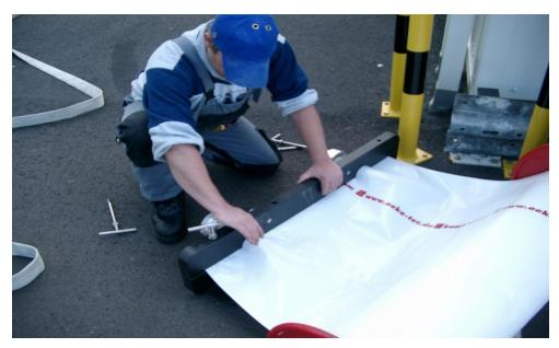
Push locking nails through the plastic material and screw hand tight until the system is secured
